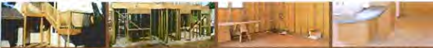
From left to right: A completed Graham Builders custom, wood-framed home. Most of the homes built by Graham Builders use wood framing. Besides wood framing, Graham Builders also uses wood trusses, plywood siding and sheathing and the T&J Joist "silent floor" system. Graham Builders uses MDF wood for much of its cabinetry.
