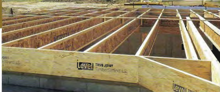
Use of engineered wood such as TimberStrand LSL truss joists shown here are a popular choice for floor and roof systems.
